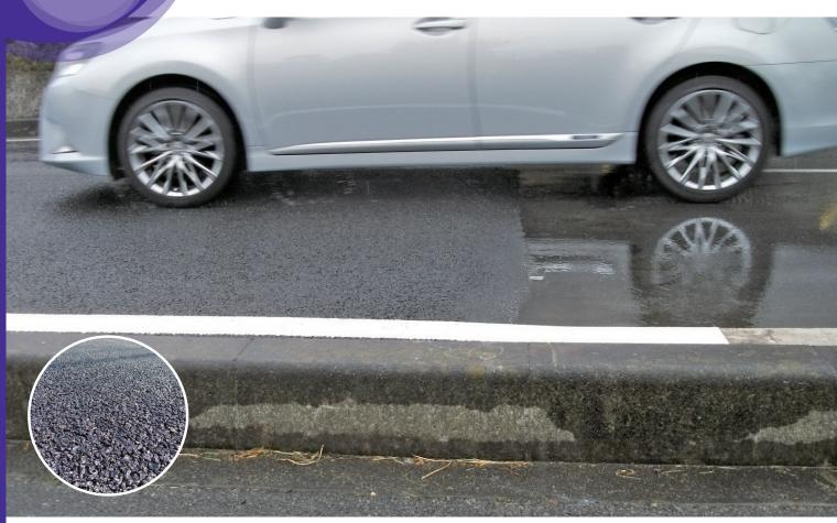
This is an inexpensive pavement for refreshing damaged asphalt pavement surfaces and improving road surface quality and extending the lifespan.
